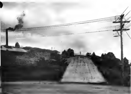
Figure 68. Ground view of a camouflaged messhall and munitions factory in Brisbane, Australia (1945). The false road continues on over the building and terminates logically at a route junction. This is an excellent example of camouflaging a permanent installation.
